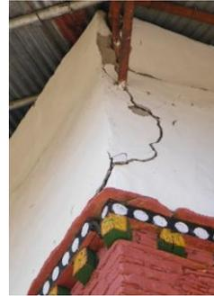
Figure 11: Flexible diaphragm action
