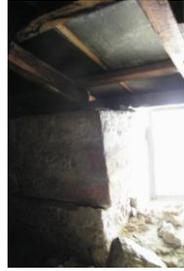
Figure 13: Collapse of random rubble stone masonry wall at top floor
