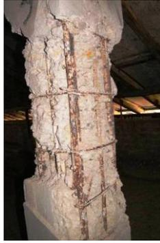
Figure 16: Spalling of concrete
