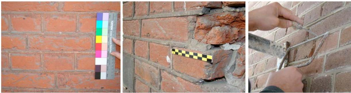
Figure 7 (left): Flemish tuck pointing of the Victor Besme phase (1880) on the facades of the inner court of the castle (© Verdonck Ann) - Figure 8 (middle): Damaged tuck pointing zone (© A. Verdonck) - Figure 9 (right): Reparation of the tuck pointing: trimming the upper edge of the ribbon with a pointing brace and knife (© A. Verdonck)
