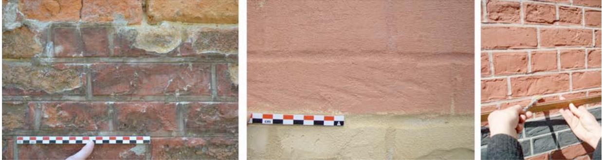
Figure 12 (left): Brickwork-imitating finish on the north façade of the farm complex: heavily polluted but well preserved zone (© A. Verdonck) - Figure 13 (middle): Restoration test strip of the base layer with sculpted joints and brick surface to simulate real brickwork (© A. Verdonck) - Figure 14 (right): Application of the red colour wash and joint painting using a brush guided by a feather-edge (© A. Verdonck)
